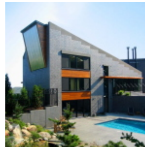
maintenance retains a fresh look building
